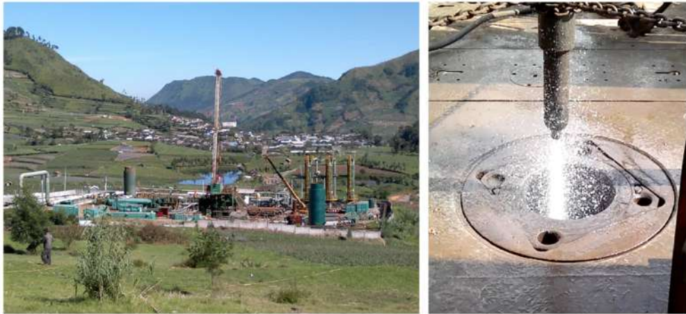
Figure 3: TFO Stimulation - Jointed Pipe Operation (Rig 550 HP) in Dieng Field
