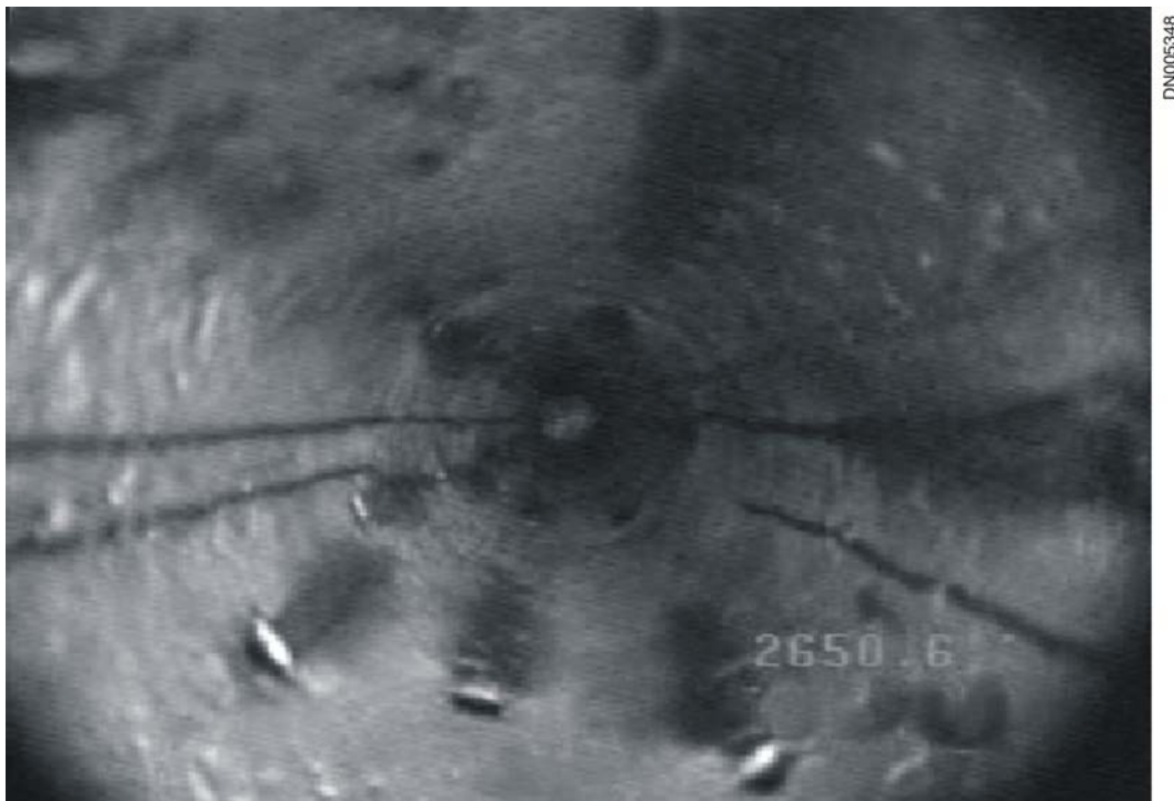
Fig. 10— Davis 1 well video after SIP treatment.
