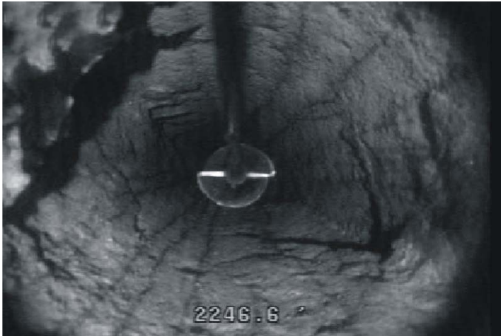
Fig. 14—Gas storage well (“B”) video after CT cleanout.
